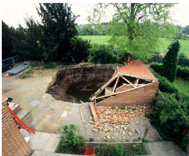
Fig. 17. One of the destructive caprock sinkholes formed by collapse over cavities in the gypsum that underlies the town of Ripon.
