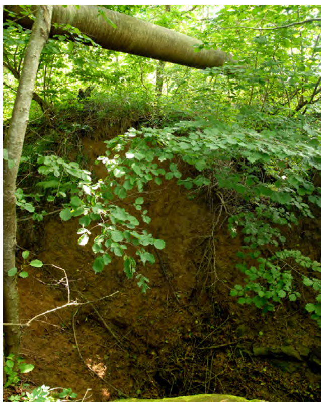
Fig. 9. An oil pipeline in Georgia is left with no support where it spans a sinkhole that developed beneath; this could have occurred soon after the inevitable drainage disturbance during construction, or subsequently owing to drainage water collecting in the trench-fill.
