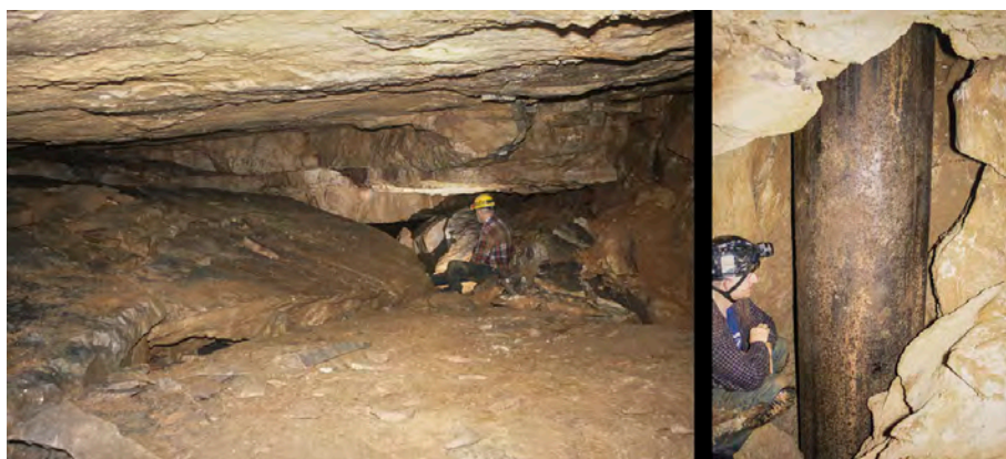
Fig. 20. Big Spring Cave, beneath the courthouse in Huntsville, Alabama. (left) Part of the width of the main passage, where beds of the nearly horizontal limestone have fallen from the roof, so that the open space is now on top of slabs stacked 5 m deep. (right) A steel-cased, bored pile that extends through the cave and debris fill, and carries its load to stable rock beneath the cave floor.
