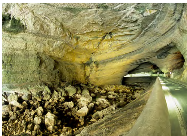
Fig. 4. Karst benefit. The cave of Mas d'Azil in the French Pyrenees, with a main road built beside the cave river to gain an easy route through a limestone ridge.
