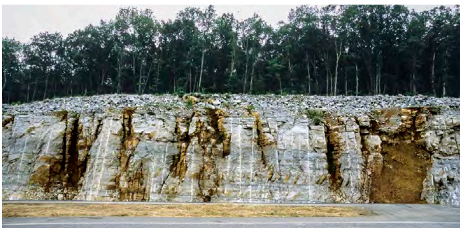
Fig. 22. Limestone exposed in a pre-split face about 5 m high alongside a road in Alabama, USA. Every few metres along the face there is a clay-filled fissure, a zone of narrow fissures or a buried sinkhole. All of these would have been potential sites for new subsidence sinkholes within the few metres of soil cover that has been removed along the crest (and replaced by the bank of limestone boulders).
